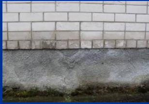
Internal thermal insulation is risky solution in cold climate: mould growth and condensation in the wall on the old wall surface
